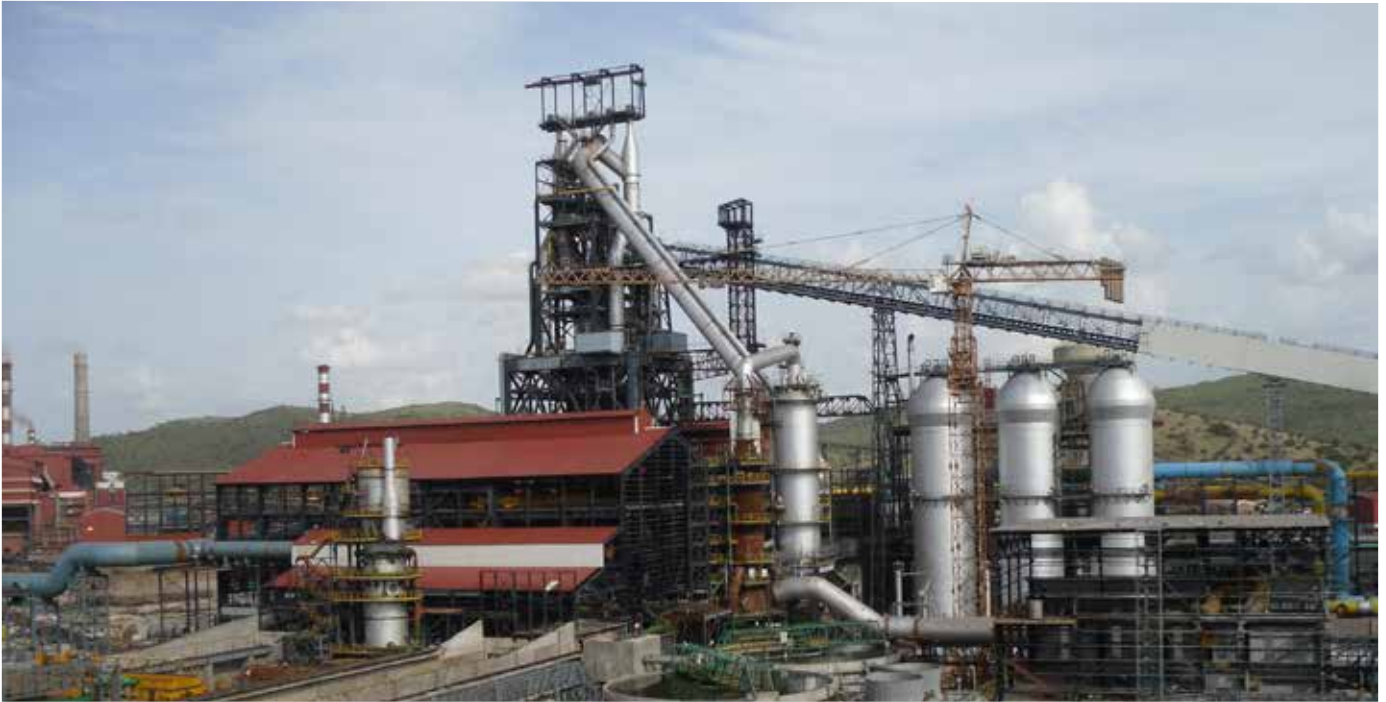
JSW Steel Limited, Toranagallu, Blast Furnace No.4
